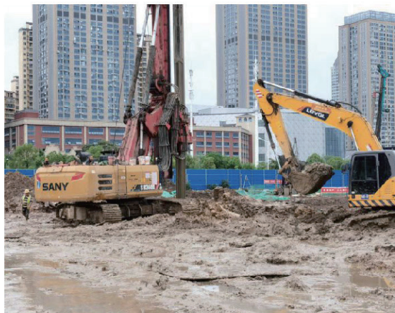
• Construction site in Wuhan Jiangxia
