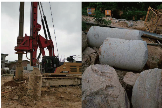
• Construction site in Fujian Putian
