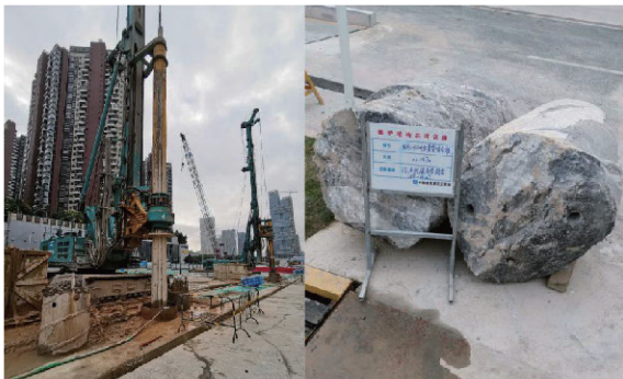
• Construction site in Shenzhen Nanshan
