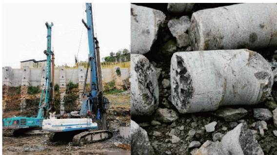
• Construction site in Chongqing
