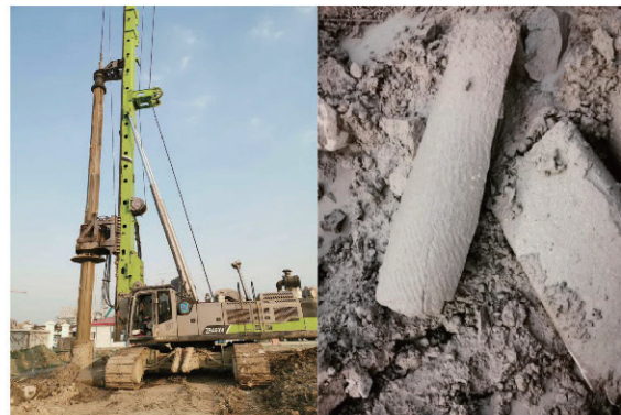
• Construction site in Suzhou Mudu
